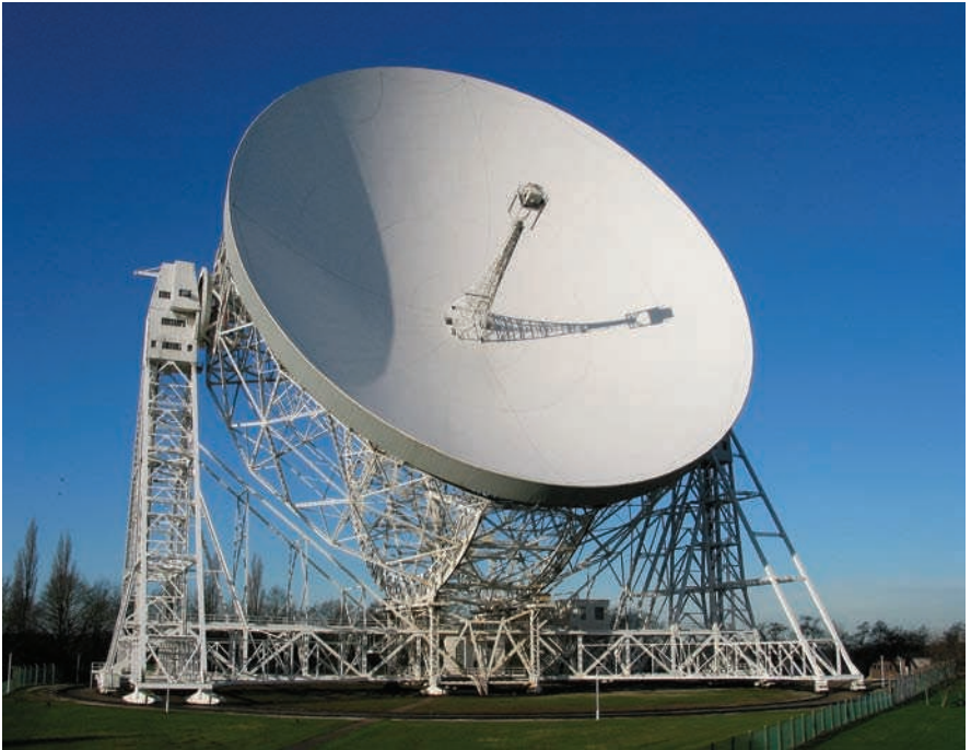
Figure 5.21 The 76-m Lovell Telescope – a prime focus design. Image: Ian Morison.
